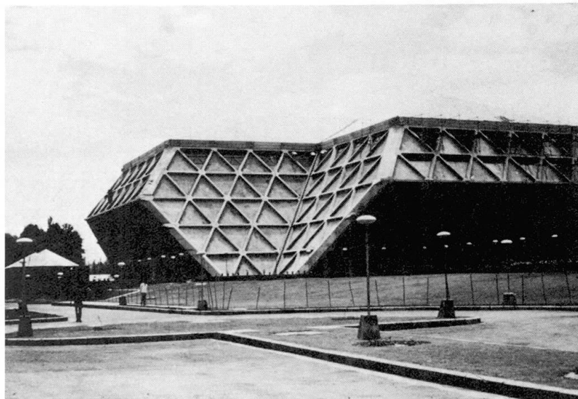
Fig. 2.5 Exterior View of Stadium
