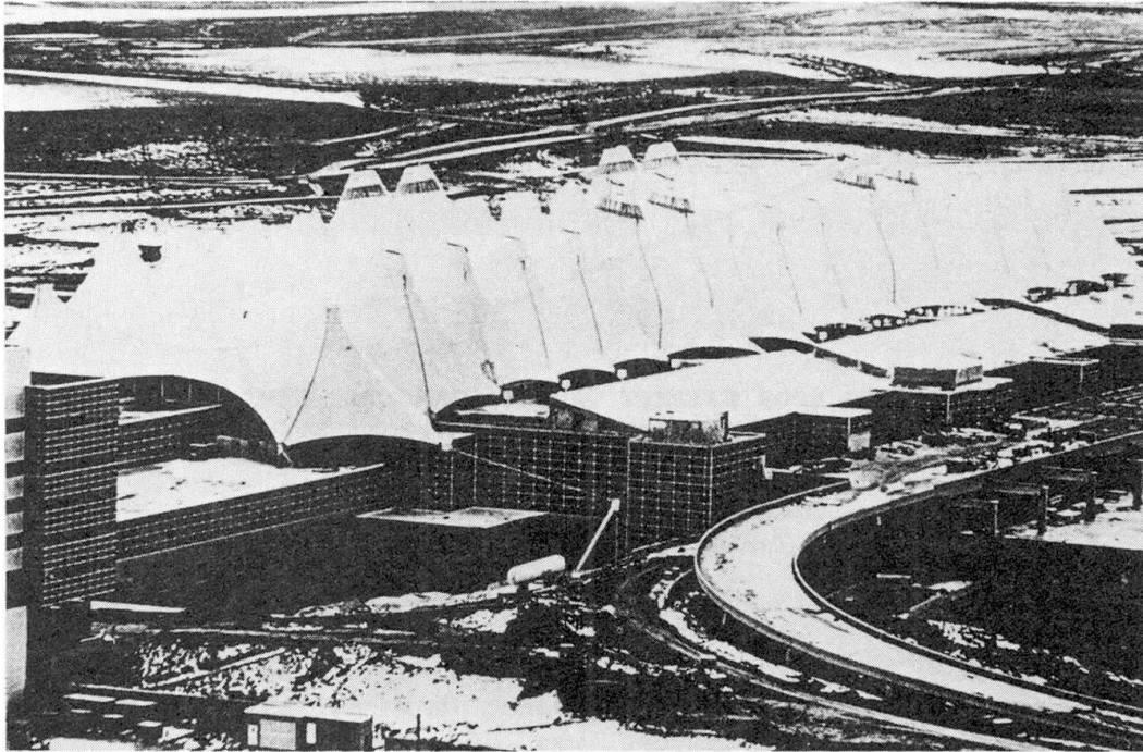
Aerial View of the Roof
