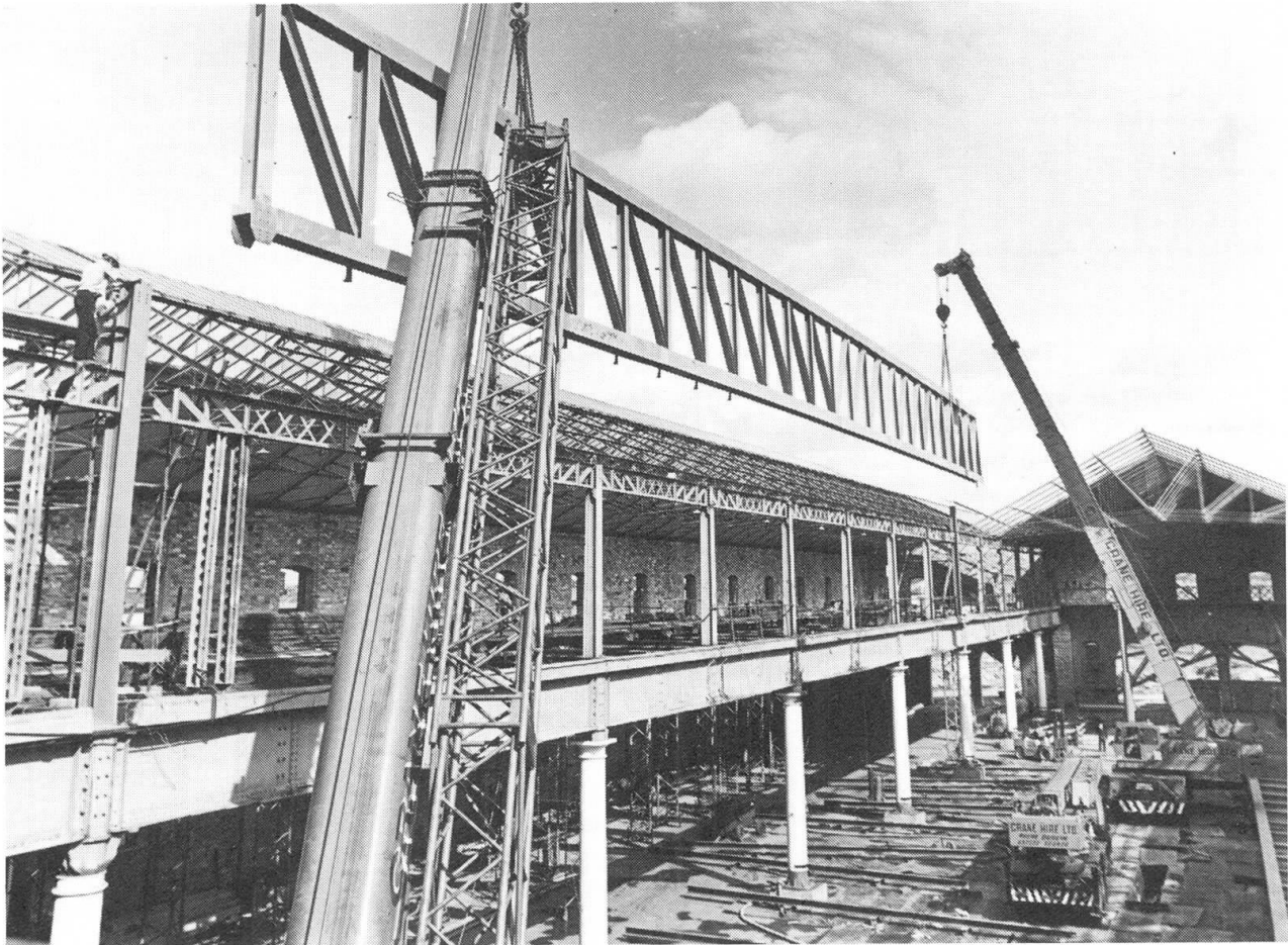
Fig.1: Erection of Main Roof Girders - Phase 1.
