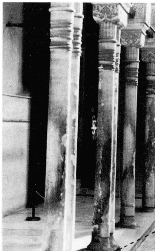
Fig. 3 Progressive reduction in height of bases, and damaged shafts according to mechanical weakness plane.
