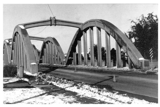
Figure 3. Circa 1930 patented Marsh encased steel through arch span at Wichita, Kansas.
