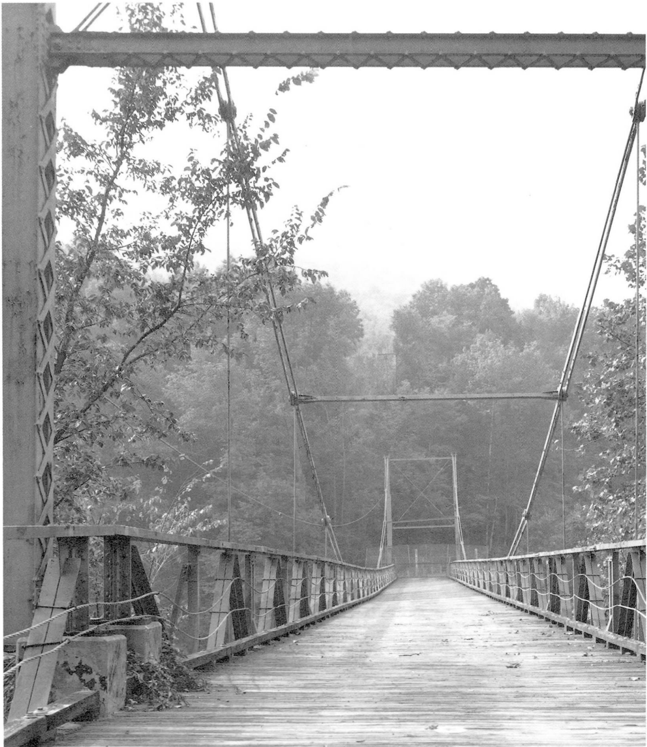
Figure 4. Ca. 1902 eyebar suspension bridge at Lordville, NY that failed and was recorded and demolished in 1986-1987.
