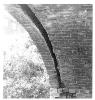
Fig 2 Crack in arch ring
