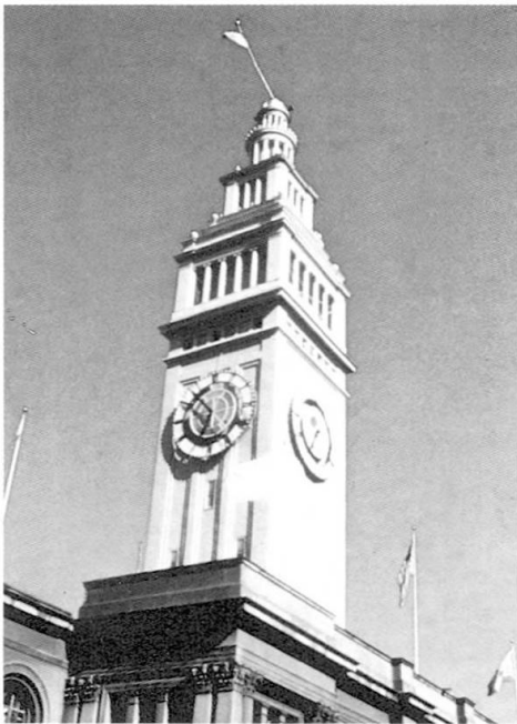
Figure 2. Photograph of Ferry Building tower after Loma Prieta earthquake with bent flagpole.
