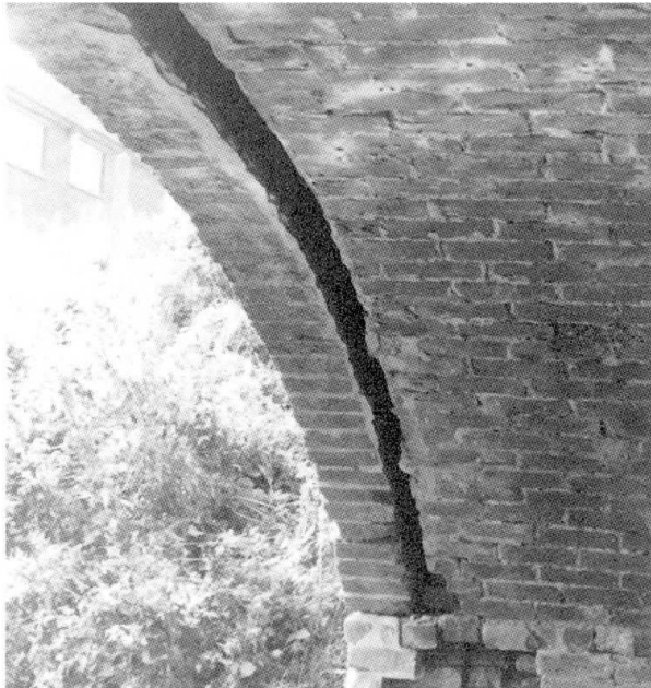
Fig 2 Crack in arch ring
