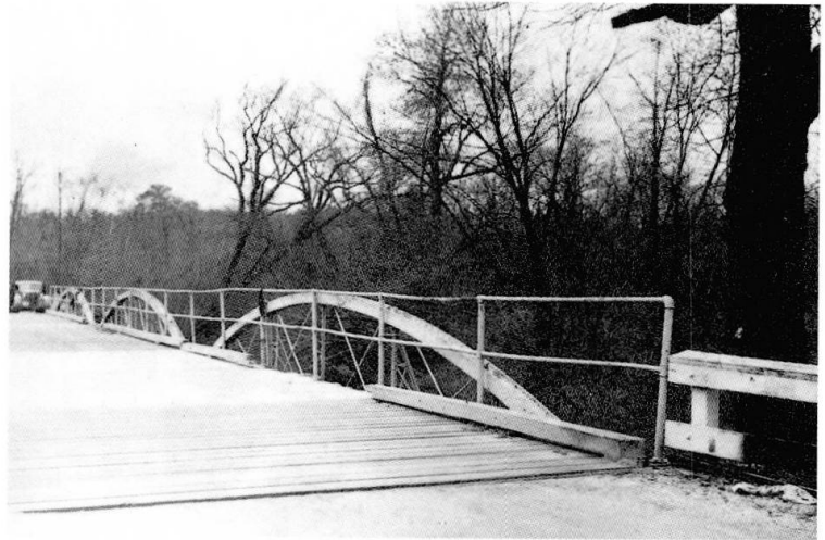
Figure 5. Ca. 1860 King bowstring truss bridge at Allenwood, NJ.
