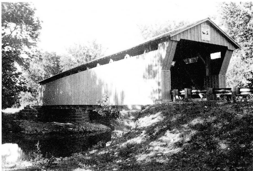
Figure 1. Rehabilitated 1887 wood truss bridge at Canal Winchester, Ohio.
