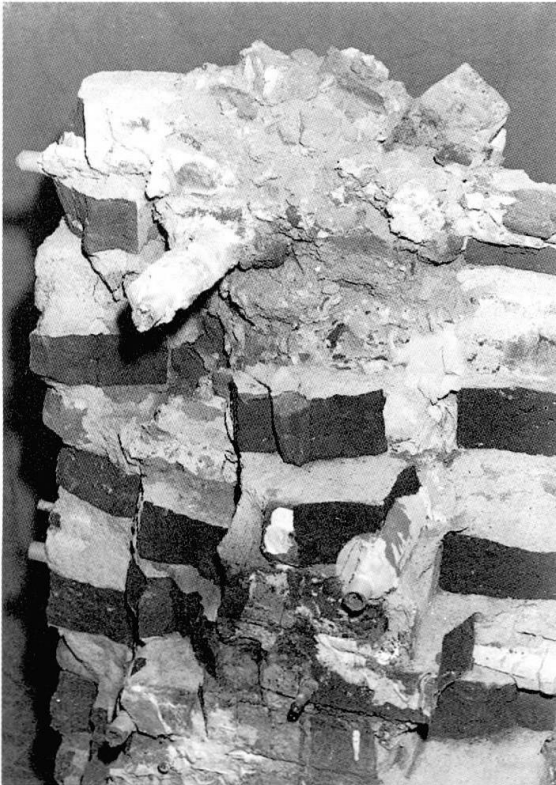
Fig. 4 Inside view of consolidated column with the connectors in place.
