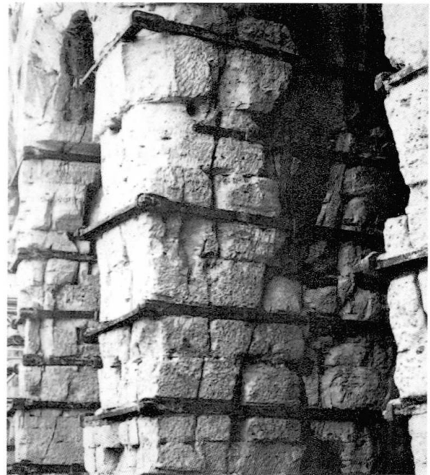
fig.8 State of the pillars on the Stern abutment side in 1979.
