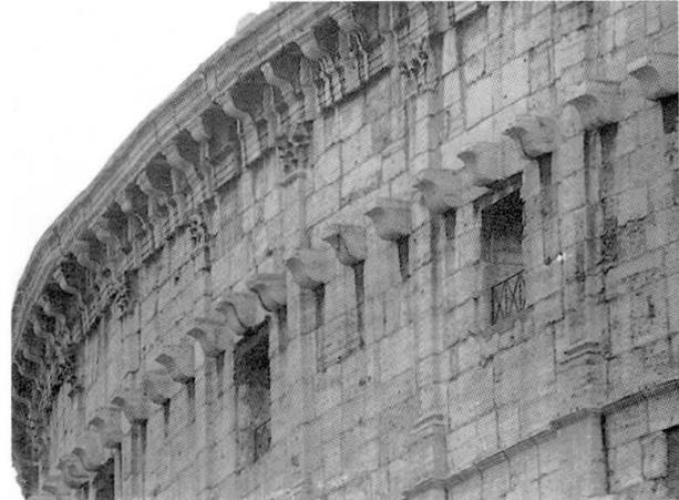
fig.6 Synusoidal deformation of the parapet.
