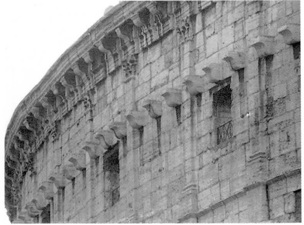
fig.6 Synusoidal deformation of the parapet.
