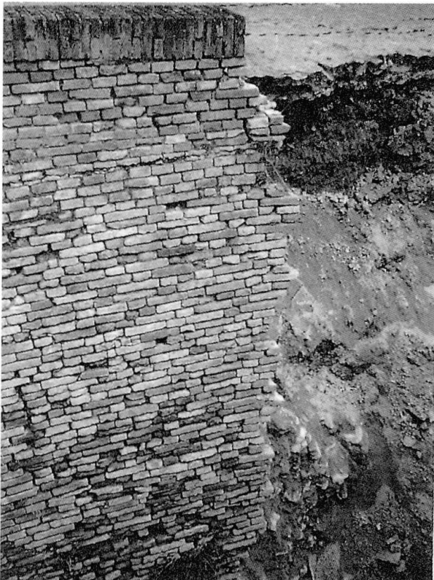
Fig. 19 A view of the Urbino walls (a), a collapsed zone where it is possible to see the poor condition of the masonry (b, c)
