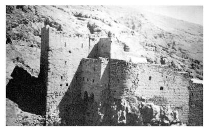
Fig. 11 Monastry of Mar Mousa in Siria: deteroration of the masonry and dangerous disintegration of the stone basement
