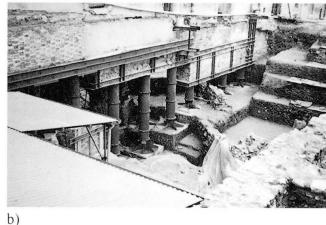
Fig. 16 The Amphiteatre of Ancona with houses built above (a) and excavation works under the foundations (b)
