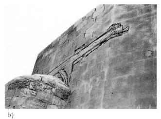
Fig. 8 Wood chains to connect the walls (a) and to counteract the thrust at the base of a dome (b)
