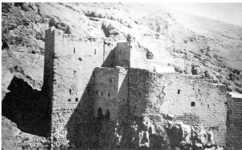
Fig. 11 Monastery of Mar Mousa in Siria: deterioration of the masonry and dangerous disintegration of the stone basement
