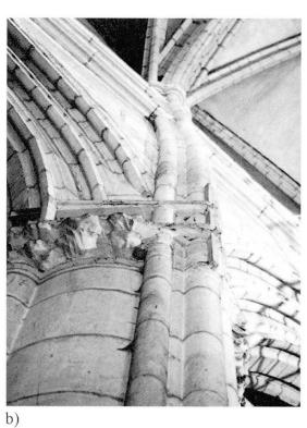
Fig. 17 The Cathedral of Vitoria in Spain (a) and the huge deformations of the columns (b)
