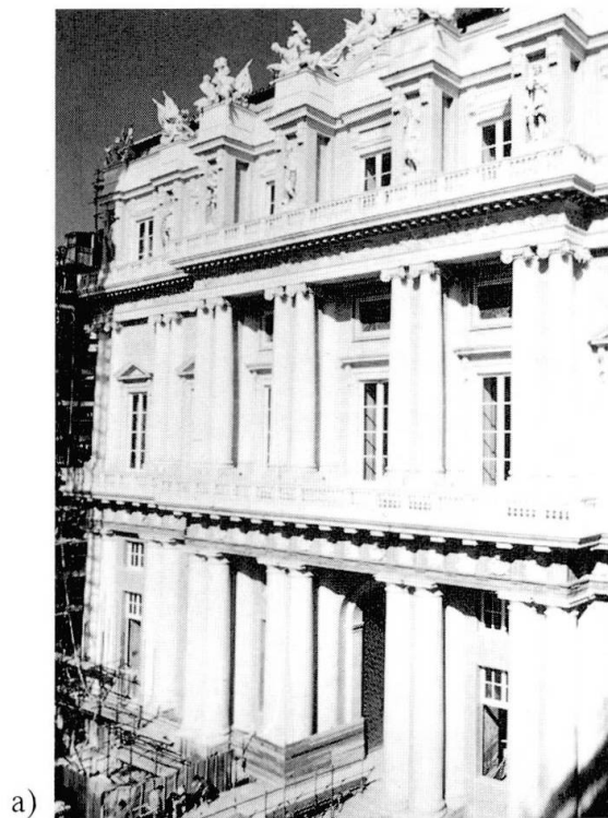
Fig. 13 The Ducal Palace of Genoa: the outward deformation of the façade (a) created by a loss in the curvature of the vault (b); the intervention (c) realized the connection between the opposite walls and support by means of springs (d) to the vault
