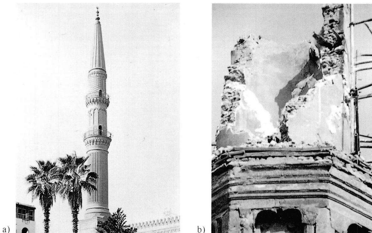
Fig. 7 Minarets in Cairo: weakness (a) and slenderness (b), often worsened by out-of-plumb
