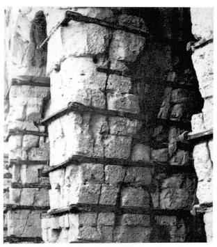
fig. 7 Spectrum response dynamic analysis fig.8 State of the pillars on the Stern abutment side in 1979.
