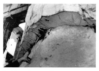
Fig. 1 Drums showing a sliding response.
