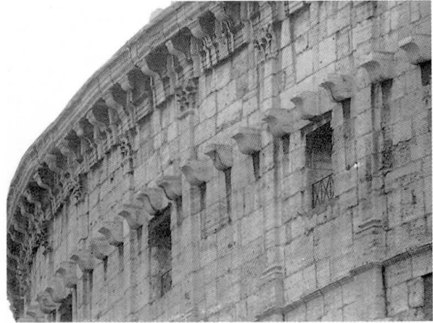
fig.6 Synusoidal deformation of the parapet.
