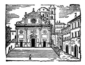
sustaining the dome. Then, L.Vanvitelli completely renovated it, consolidating all foundations, dismantling the whole dome and replacing the old bell-tower (both still appearing in the engraving).
