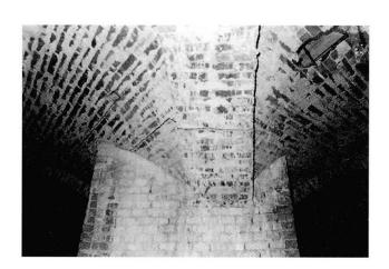
Fig. 4 - Fissures in the the 12 cm thick vaults on the underground level.
