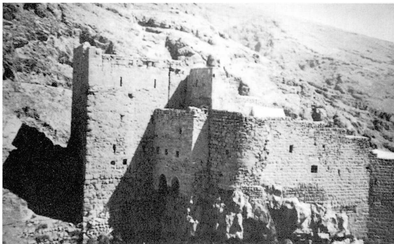
Fig. 11 Monastery of Mar Mousa in Siria: deterioration of the masonry and dangerous disintegration of the stone basement
