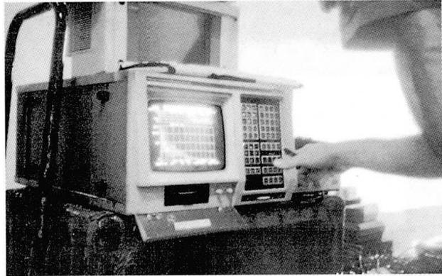
Fig. 6 Impact Echo Data on Field Computer
