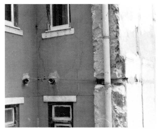
Fig. 2: Damaged masonry wall due to demolition of an adjoining building
