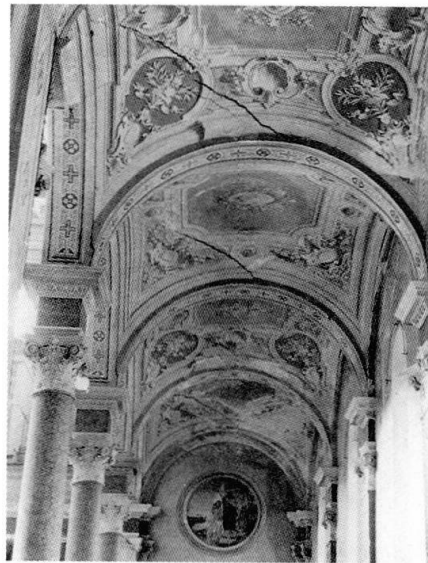
Fig. 3 - Fissures in the thin vaults of the side aisles.
