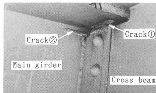
Photo 3 Fatigue cracks occurring at cross-beam connection
