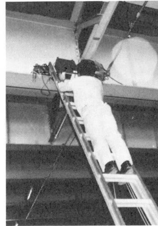
Photo 2 Initial setting of histogram recorder in field
