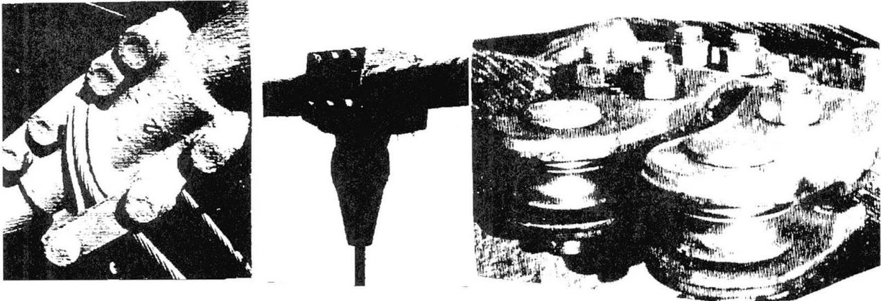
Fig.2 Clamped boundary-cables
