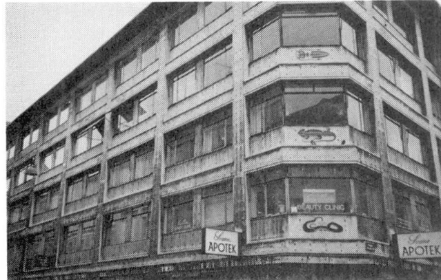
Figur 4: Miscoloured facade due to dirt and soot
