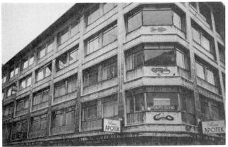
Figur 4: Miscoloured facade due to dirt and soot
