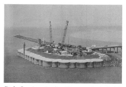
Fig. 5: Protection against ship collisions, supporting the foundation works of the North pylon (Winter 90-91)
