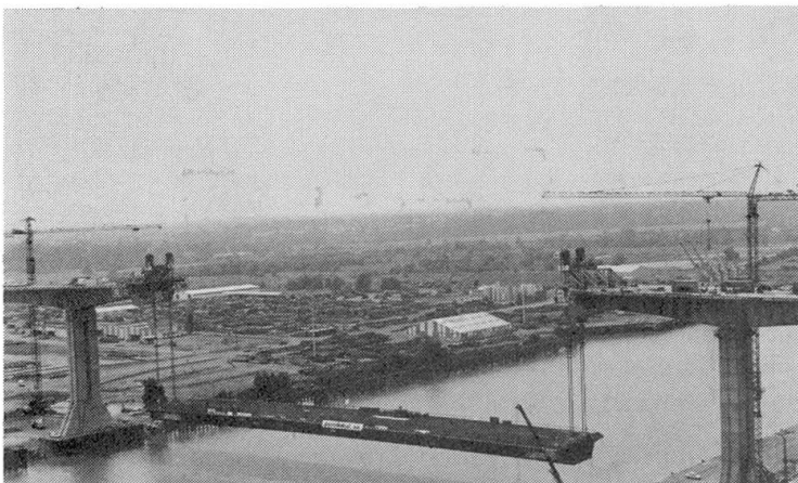
Figure 7: The Cheviré Bridge: the steel isostatic span is now lifted from the two concrete cantilevers (photo G. Forquet)
