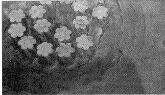
Fig. 3: Crack along strand bundle
