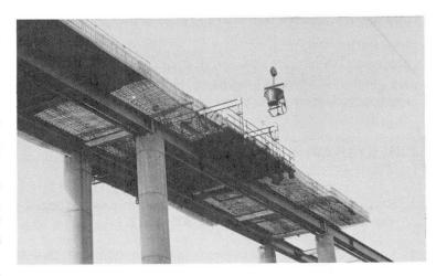
Figure 9: The bridge over the River Rance; concreting the top slab (photo G. Forquet)
