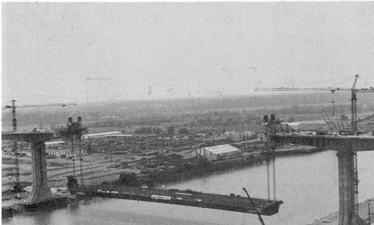
**Figure 7:** The Cheviré Bridge: the steel isostatic span is now lifted from the two concrete cantilevers
