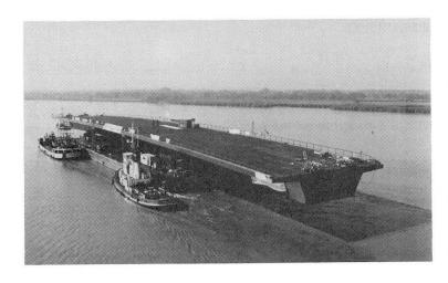
The Cheviré Bridge. The steel isostatic span on its Figure 6: barge during transport (photo G. Forquet)
