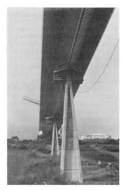
Figure 3: The Val de Maupré viaduct, at Charolles, during erection (photo G. Forquet)
