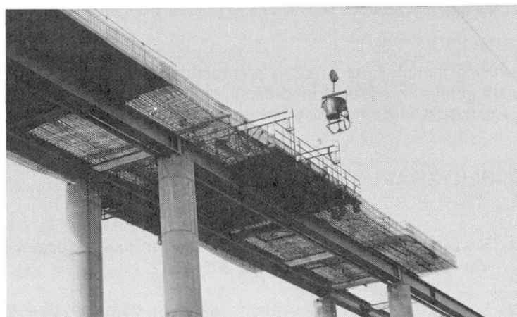
Figure 9: The bridge over the River Rance; concreting the top slab (photo G. Forquet)
