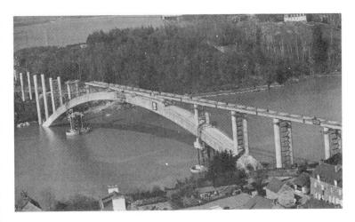
Figure 8: The bridge over the River Rance; the steel structure during erection (photo G. Forquet)
