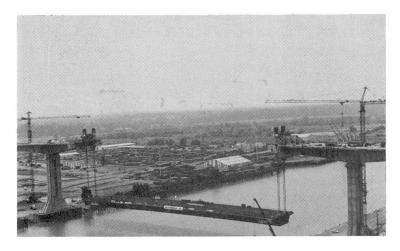
Figure 7: The Cheviré Bridge: the steel isostatic span is now lifted from the two concrete cantilevers (photo G. Forquet)
