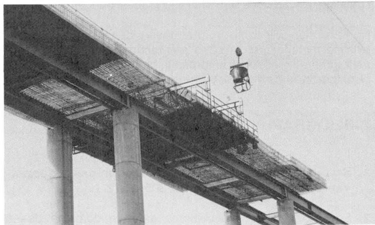
**Figure 9:** The bridge over the River Rance; concreting the top slab
