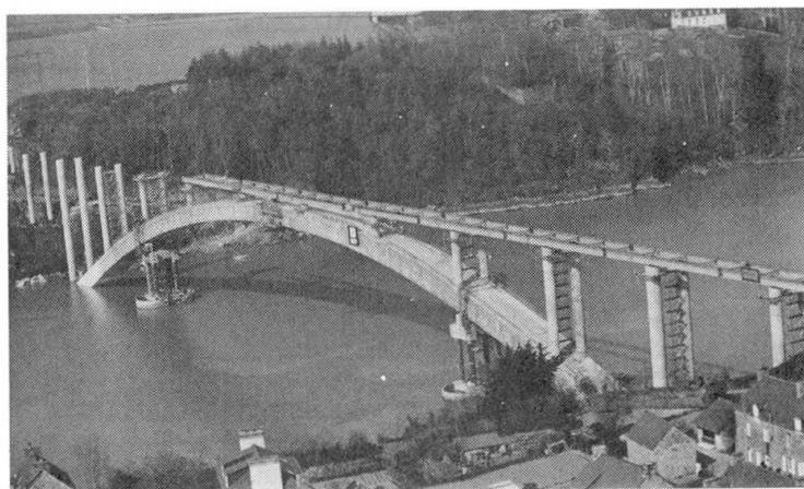
Figure 8: The bridge over the River Rance; the steel structure during erection (photo G. Forquet)
