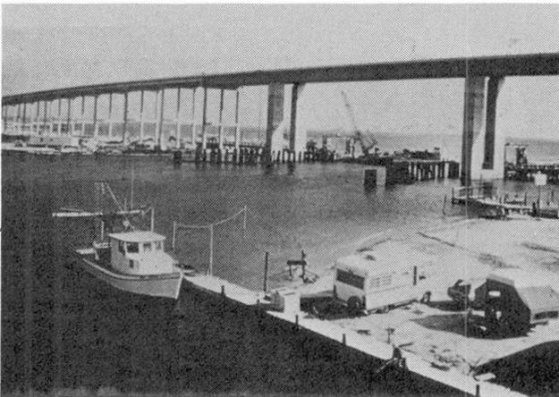
The precast segmental concrete bridge located at Corpus Christi Texas was the first of its kind in the United States. The construction method was precasting by the long line method and erecting by balanced cantilever with the segments being delivered with barge mounted cranes. It represented a modest beginning as related to the size of project. The structure consisted of three spans of 31m - 62m - 31m. [1]
