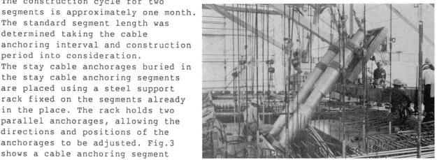
Fig. 3 Construction of stay cable anchoring segment
