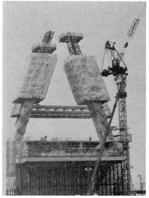
Fig. 2 Tower construction by climbing forms
