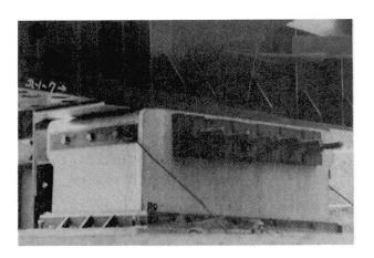
Fig. 10 Temporary shoe for launching
