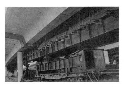
Figure 11 - Curved structure of the South Bridge Span-by-span assembly of precast segment "PRK".
