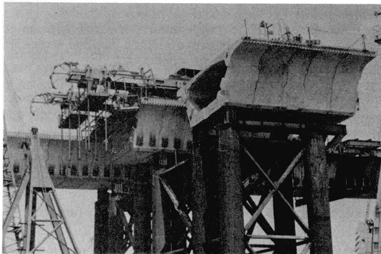
Figure 10 - South Bridge - Segmental in progress. One typical precast segment "K" placed in the superstructure.
