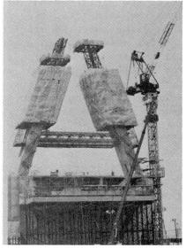
Fig. 2 Tower construction by climbing forms
