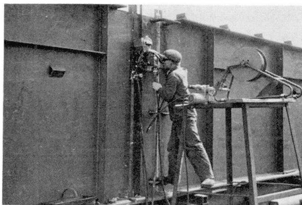
**Fig. 6** Device for submerged-arc welding of vertical joints.
