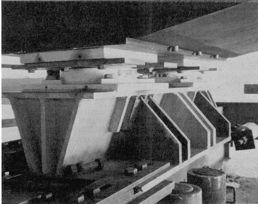
**Figure 3** Details of launching carriage and bearing assembly showing bearings; bolted steel plates to inhibit translation of bridge relative to bearings; welded launching carriage; and (bottom left) steel-reinforced Teflon-coated neoprene pad projecting from beneath the launching carriage.
