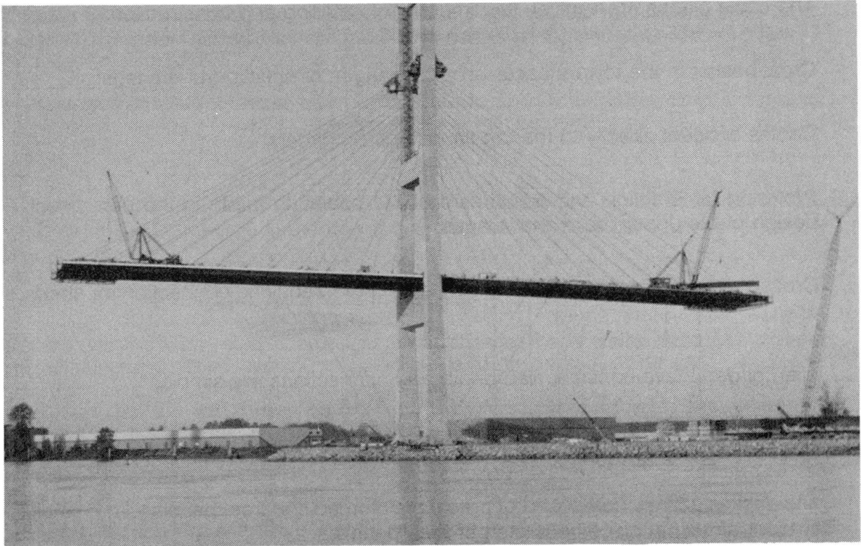
Figure 6. Alex Fraser Bridge under construction.
