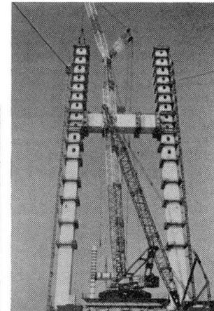
Fig.4 Tower Construction by Block System
