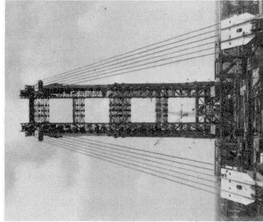
Photo 2 Side View of Temporary Cable-Stayed Tower
