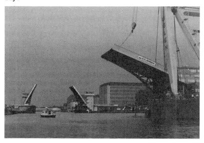
The bridge is a double leaf bascule bridge from 1939 with a bascule span of 35 m (free navigation clearance) and a deck width of 27 m.
