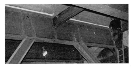
Fig. 1 Grout Bags Being Pressurised
