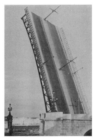
Fig. 2 The single-leaf bascule bridge
