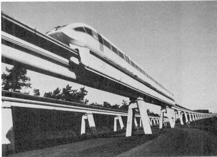
Fig. 1 Concrete guideway for the TRANSRAPID Test Facility Emsland, 1st construction phase with MagLev vehicle
