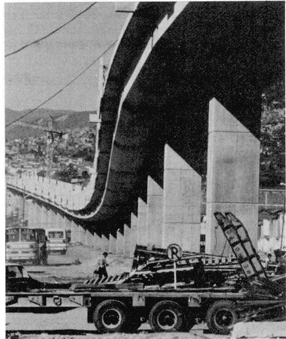
Fig. 7 Metro Medellin, elevated line under construction
