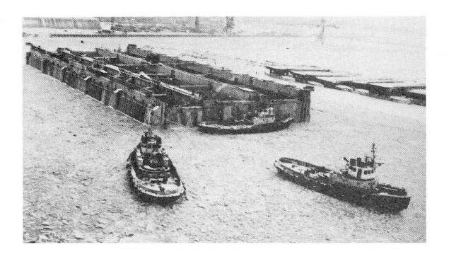
Fig.5 Transporting of floating units for sluicegates
