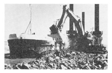
Fig.3 "Osvag"floating excavating machine
