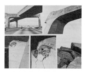
Fig. 1 Outrigger bent joint damage
