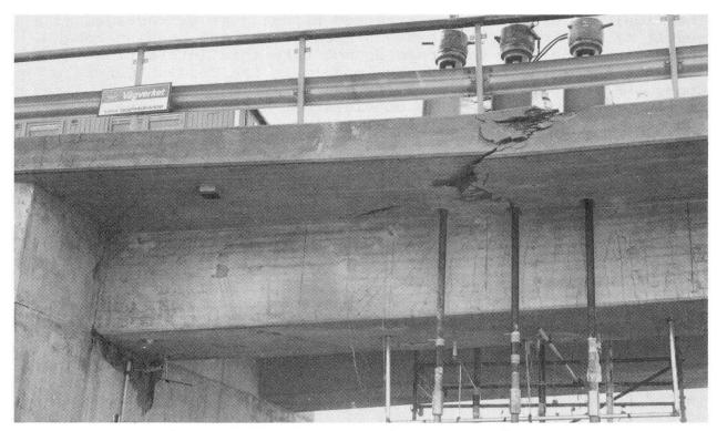
Fig. 7 Failure in the prestressed bridge. Cracking, support failure and concrete compression failure at the top of the loading section can be seen.
