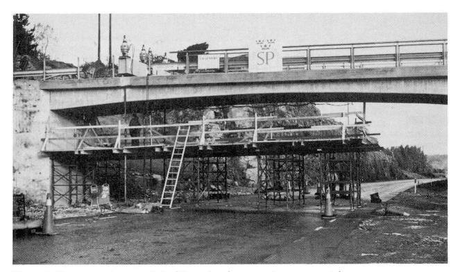
Fig. 1 Non-prestressed bridge during test preparation.
