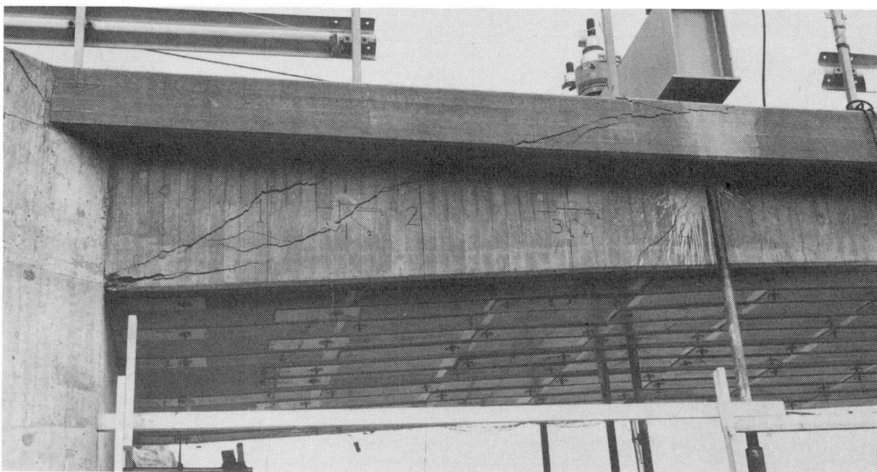
Fig. 6 Shear failure in the non-prestressed bridge
