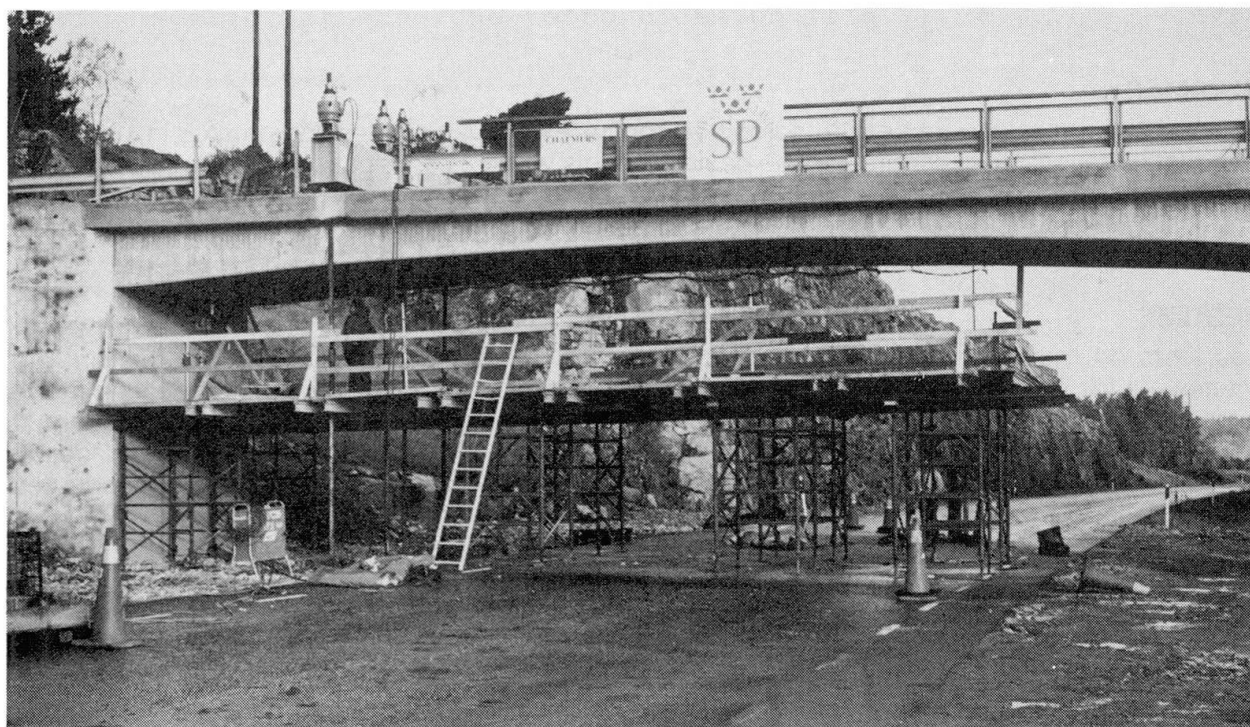
Fig. 1 Non-prestressed bridge during test preparation.
