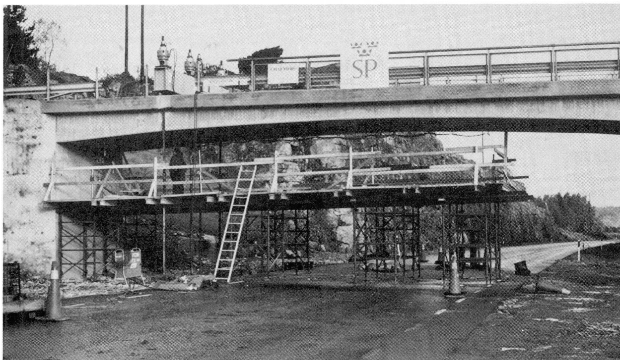
Fig. 1 Non-prestressed bridge during test preparation.
