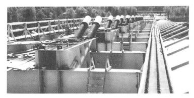
Picture 5. Cable anchoring structures, studs
