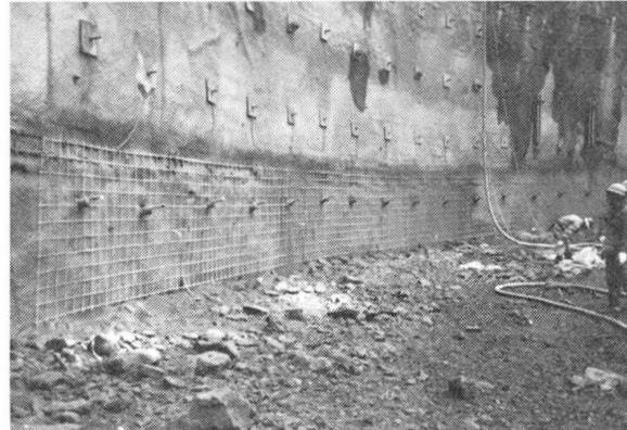
Fig. 2 Reinforcing grids for shotcrete
