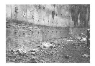
Fig. 2 Reinforcing grids for shotcrete
