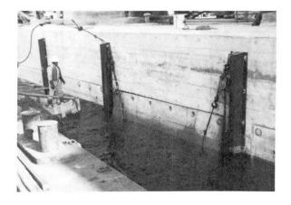
Fig. 5 Installing work of fender plate
