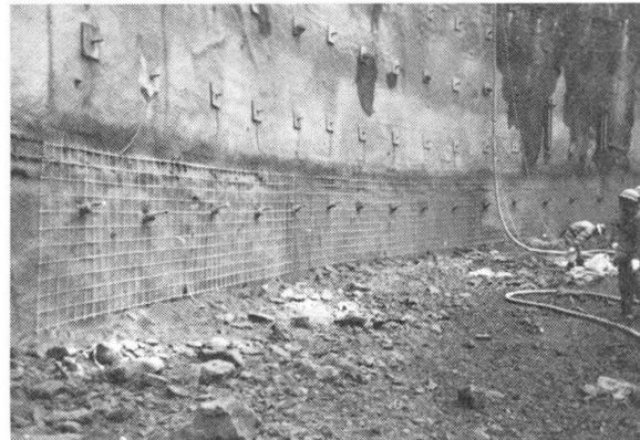
Fig. 2 Reinforcing grids for shotcrete
