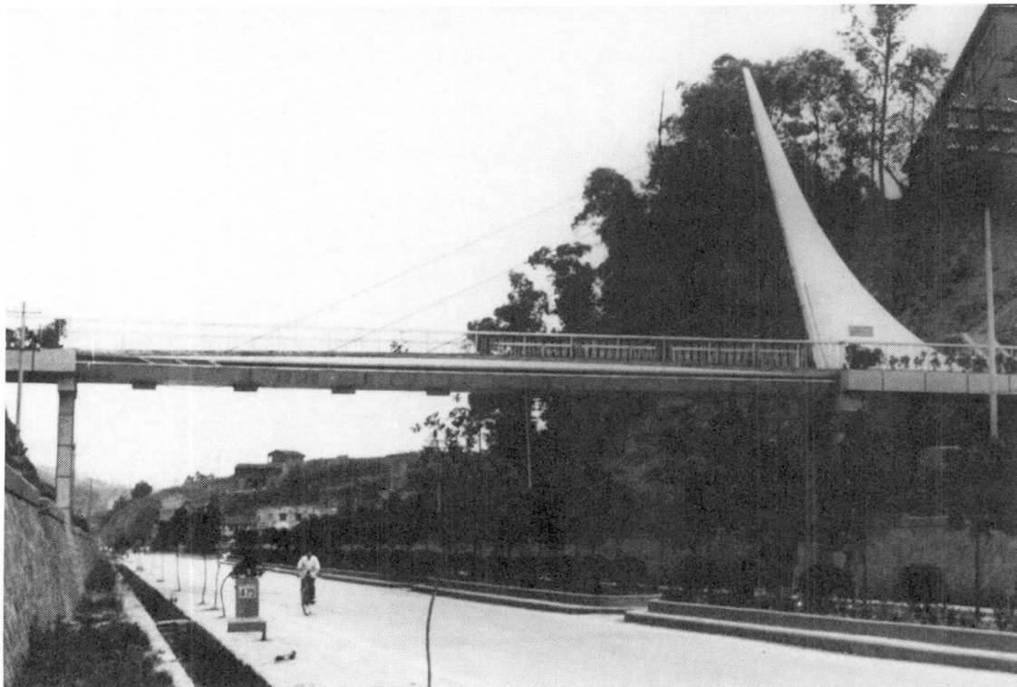
Fig. 1 GRP Pedestrian Cable Stayed Bridge
