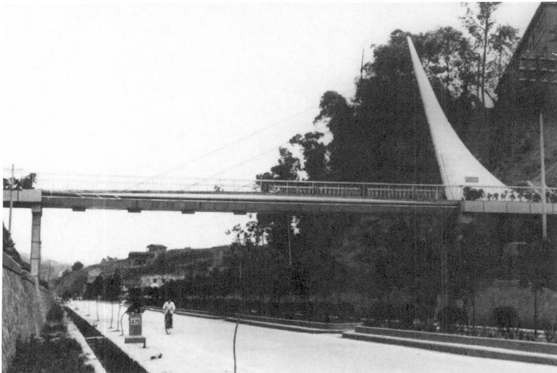
Fig. 1 GRP Pedestrian Cable Stayed Bridge
