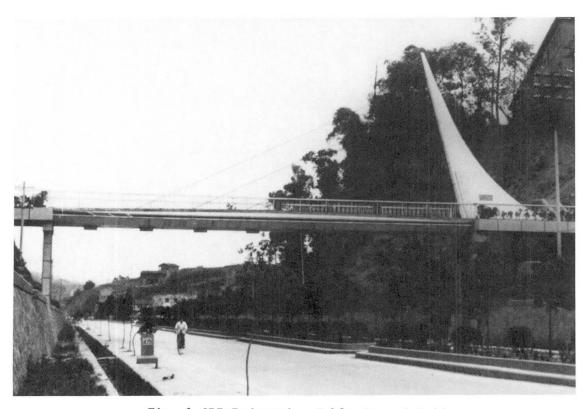
Fig. 1 GRP Pedestrian Cable Stayed Bridge
