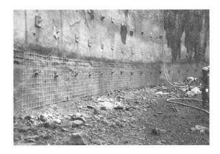
Fig. 2 Reinforcing grids for shotcrete
