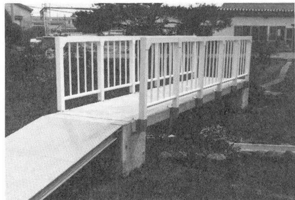
Fig. 11 Prestressed concrete pedestrian bridge
