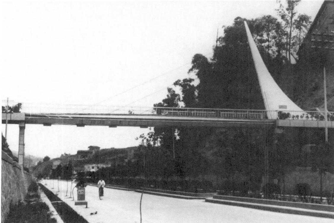
Fig. 1 GRP Pedestrian Cable Stayed Bridge
