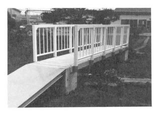
Fig. 11 Prestressed concrete pedestrian bridge
