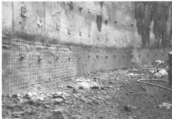
Fig. 2 Reinforcing grids for shotcrete
