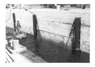
Fig. 5 Installing work of fender plate
