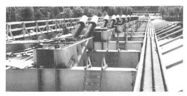
Picture 5. Cable anchoring structures, studs
