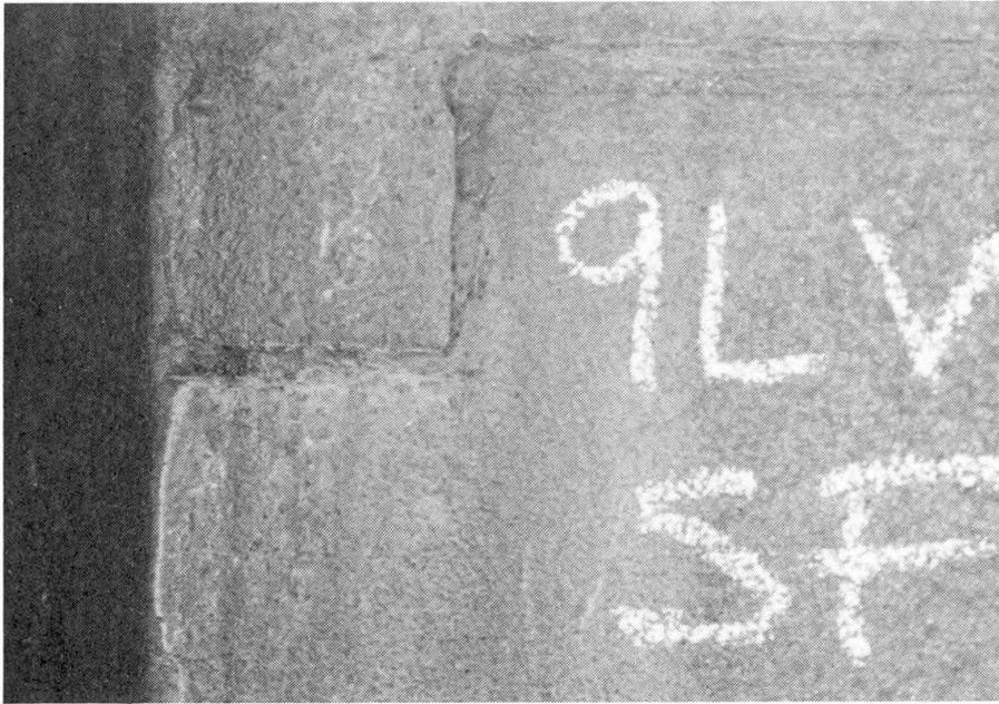
Fig. 9 Cracks at the Cope Closure Plates of a Box Beam
