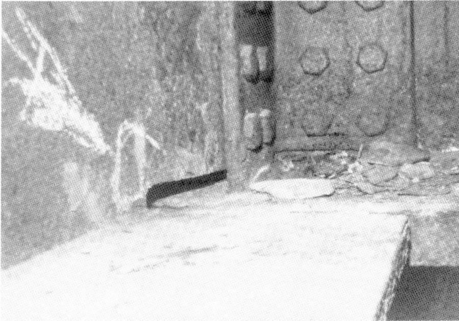
Fig. 5 Vertical and Horizontal Fatigue Cracks at Bottom Web Cope
