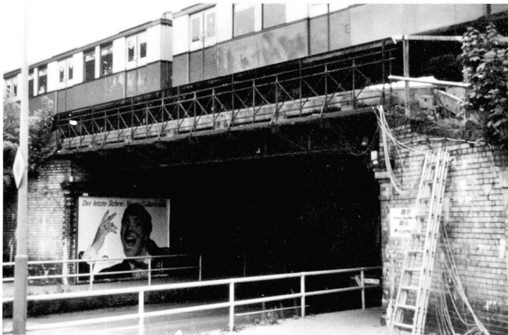
Figure 1. Steel bridge of the Berlin Metropoli- tan, built in 1898, replaced 1988
