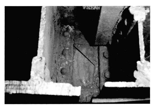
$\underline{\text{Fig. 4}}$  Connection between transverse girder and main girder, crack in web plate
