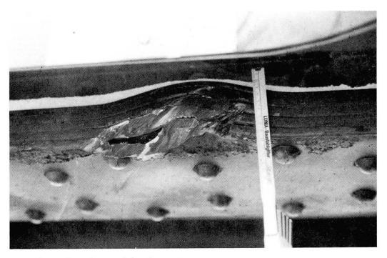
Fig. 1 Bridge damaged by impact
