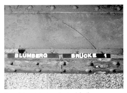
Fig. 7 Points of fracture of main girder I
