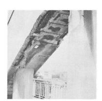
Fig.2. Corrosion of reinforcement and spalling of concrete on various elements of the bridge
