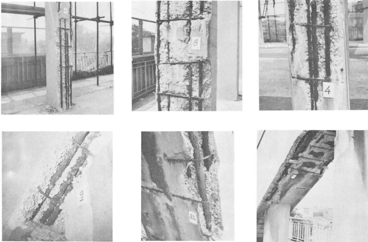
Fig.2. Corrosion of reinforcement and spalling of concrete on various elements of the bridge
