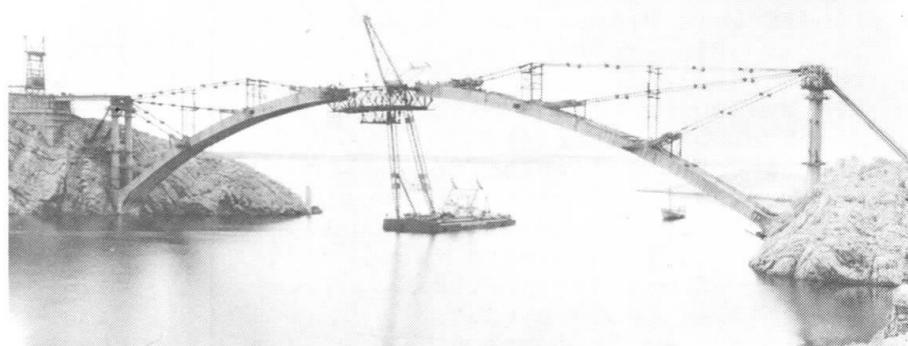
Fig 2. Reinforced concrete arch of Pag Island bridge during construction
